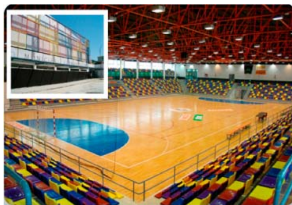
MUNICIPAL INDOOR SPORTS CENTRE "FERNANDO ARGÜELLES"
